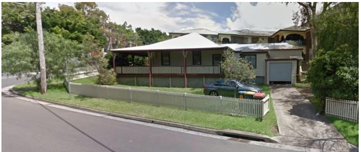
Figure 6 Heritage item – 10 Cowell Street, Gladesville Source: Google Street View
